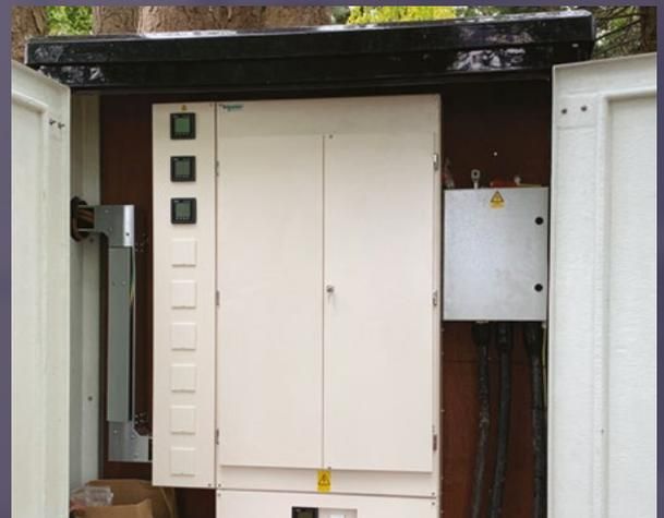
▲ AFTER: The new MCCB Panel board being installed within the new GRP enclosure.
