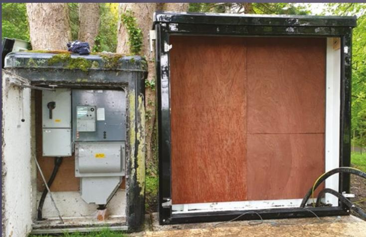
▲ BEFORE: The newly built GRP enclosure (right-hand side) to house the new MCCB Panel board. Note: the old existing enclosure is on the left-hand side.
