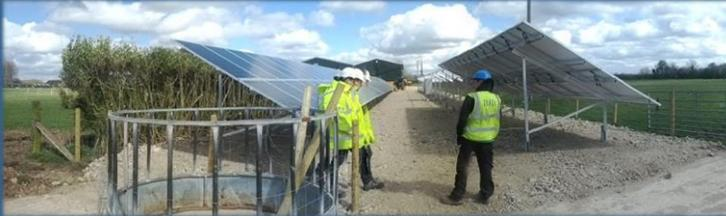
The 50kWp system at Northfield Orchard Farm provides evidence of the capability to design and install ground based PV arrays. This included assisting the client with planning and grid connection requirements
